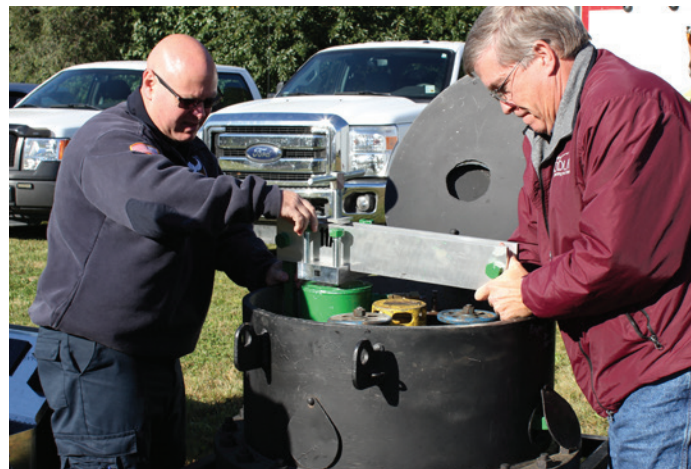
At this station, trainees practiced installing a Chlorine C-kit.
