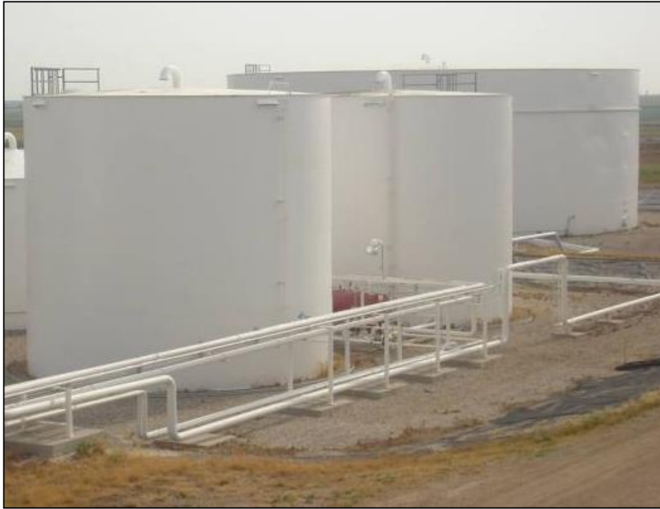
Figure 5.1: Internal Floating Roof Storage Tank
