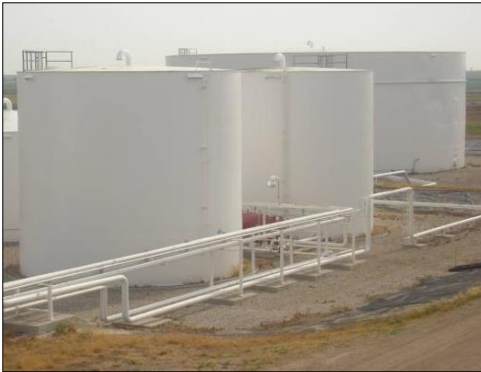
Figure 5.1: Internal Floating Roof Storage Tank
