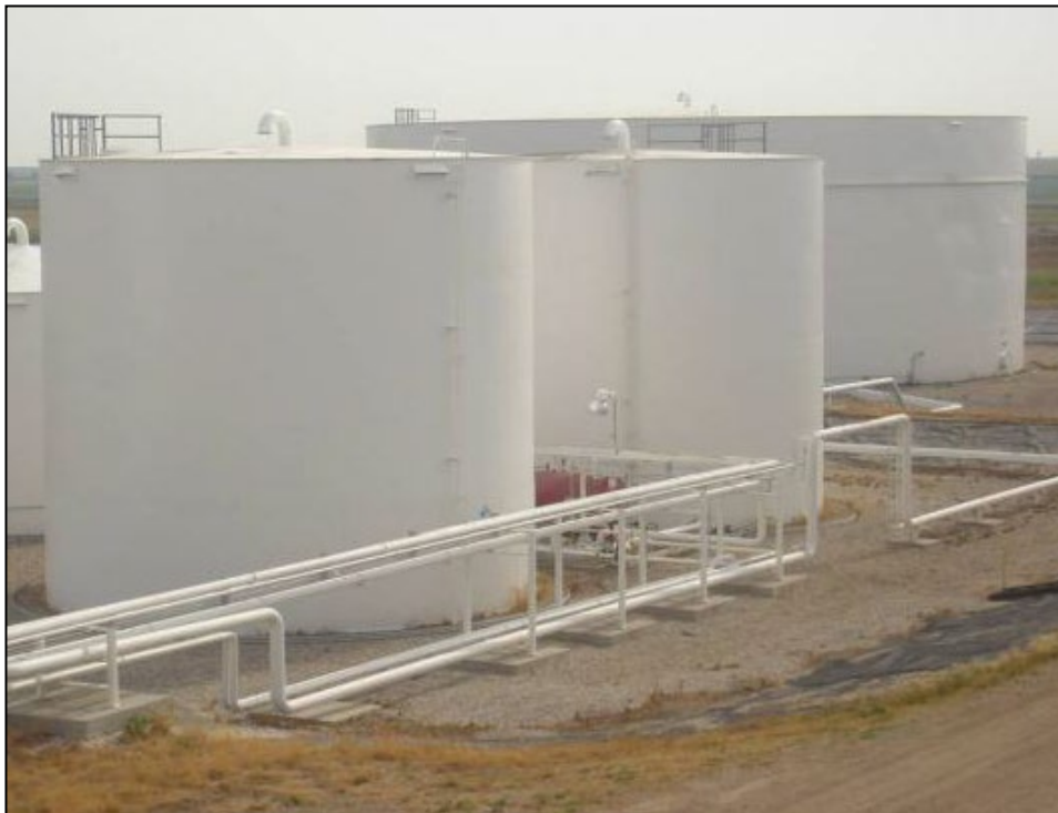
Figure 5.1: Internal Floating Roof Storage Tank
